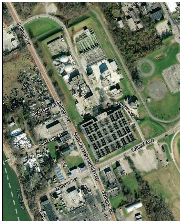
Figure 2. The Little Miami WWTP.
